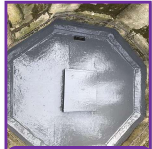
Two Tower Repair £12,374
